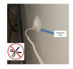
Once the probe is removed from the glycol bottle, gently slide the probe out of the \*auxiliary port in your unit. *Please note: the probe cable may be ran through the door.*
